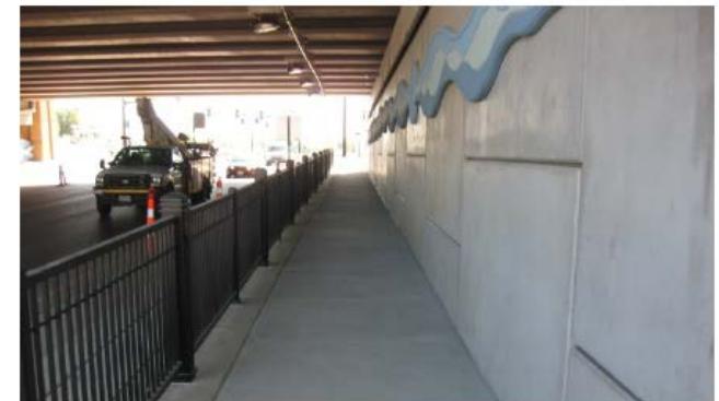
Exhibit 3-3. Outside walkway at Dorsett Road (Maryland Heights, MO). (14)
