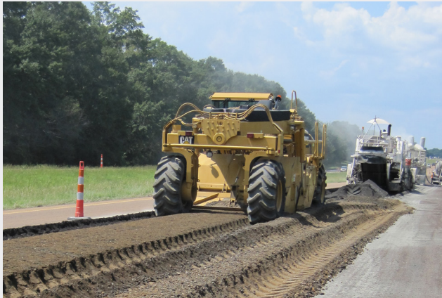
Cold in-place recycling involves pulverizing old pavement and constructing new pavement in series.
