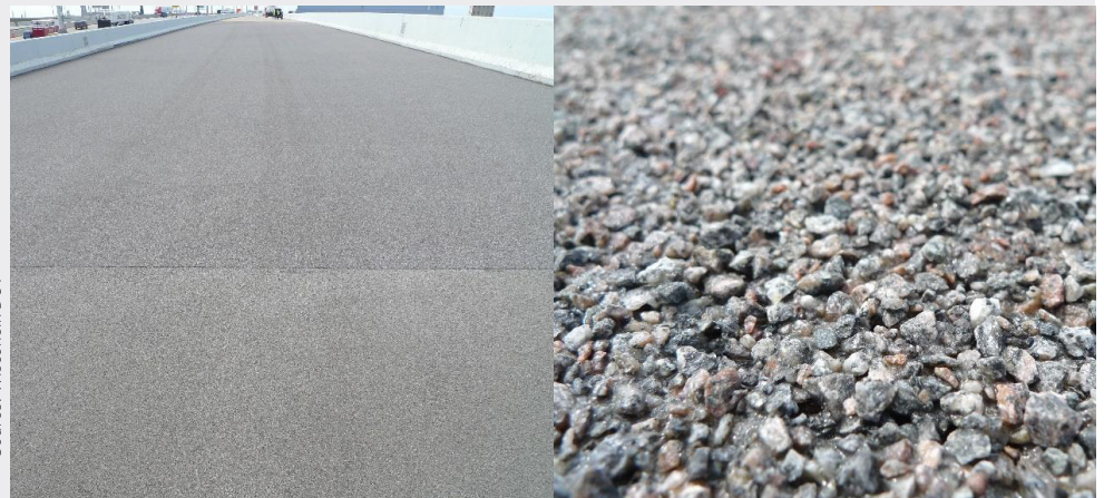
Thin polymer overlays provide skid and corrosion resistance to new bridge decks.
