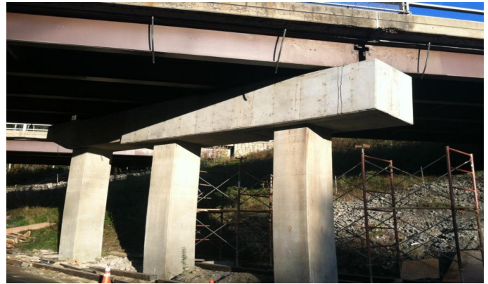
Repairs studied include those made to bearing seats and piers on an Interstate 89 bridge in Richmond, Vermont.
