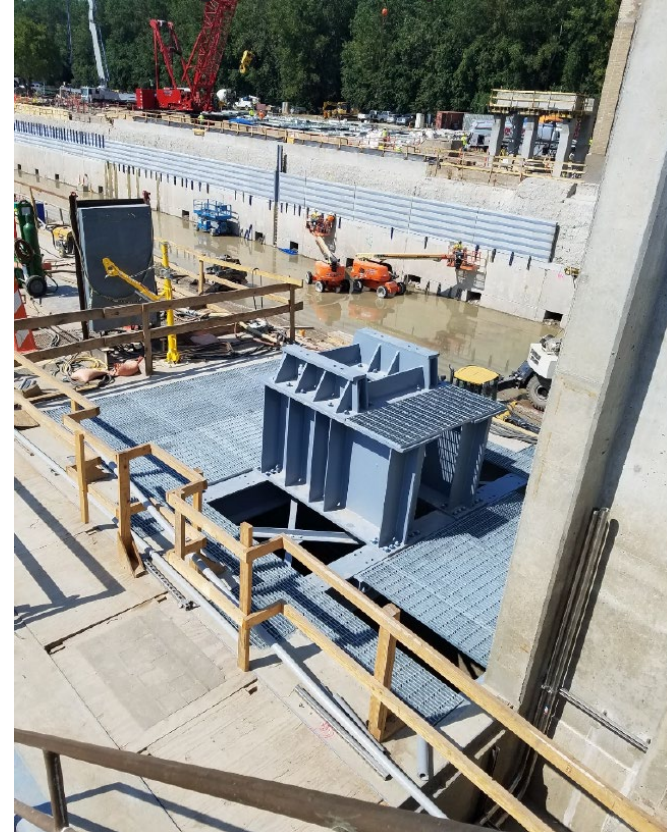
New gate machinery base
