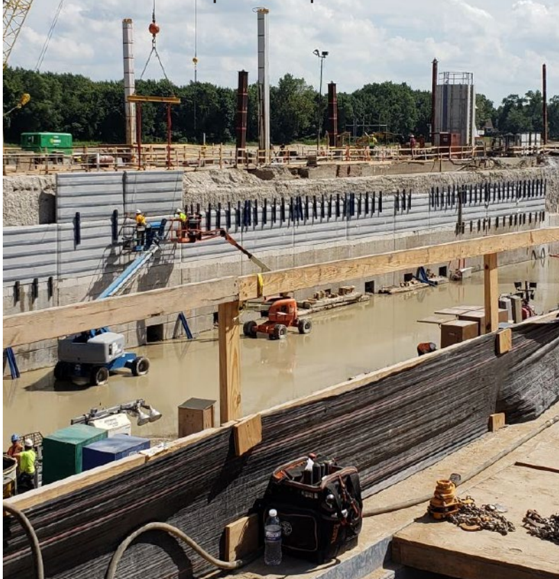
Vertical concrete pre-cast panel installation
