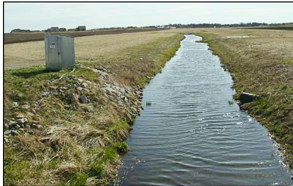
Kickapoo Creek at CR 2100E Bridge
