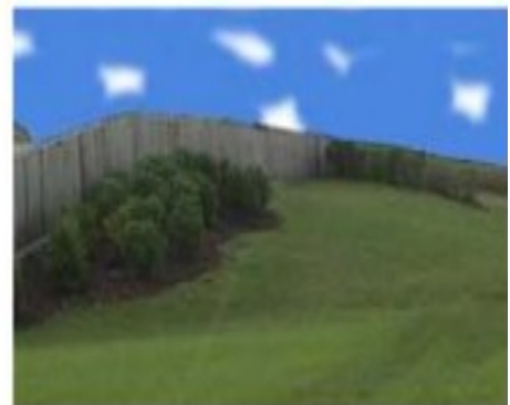
Combination of Noise Walls and Earth Berm
