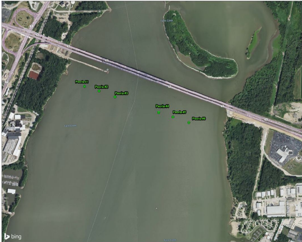
Figure 42. Aerial Photo. Sample locations at McCluggage Bridge.
