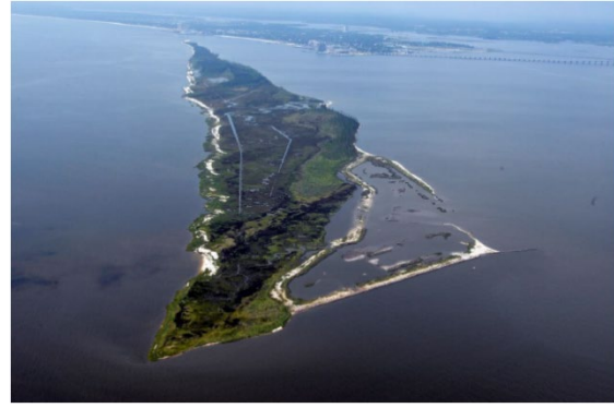
Figure 4. Post-Hurricane Katrina showing storm damage (December 2005) (Roth et al., 2012).
