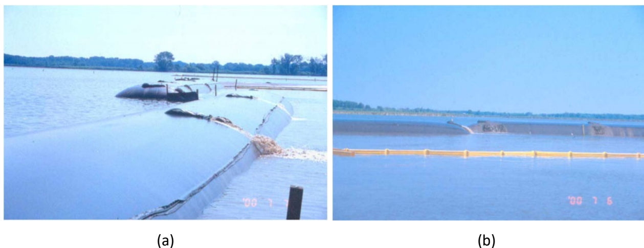
Figure 9. Photos. Geotubes in Grass Lake: (a) geotubes almost full of sediment and (b) geotubes and silt screen in the foreground (Bhowmik & Demissie, 2001).
