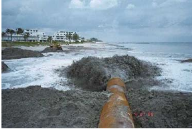
Figure 10. Photo. Beach nourishment using dredged material in the USACE Galveston District (Collins et al., 2015).
