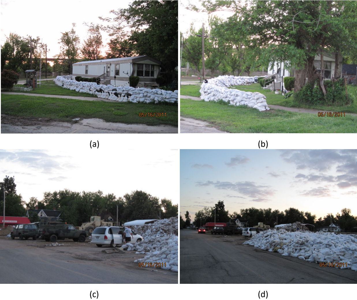
Figure 29. Photos. Photographs of (a) and (b) sandbags to protect a residence and (c) and (d) a public sandbag filling area in Ohio when Ohio River flooding occurred in 2011 (Photos taken by T. D. Stark).
