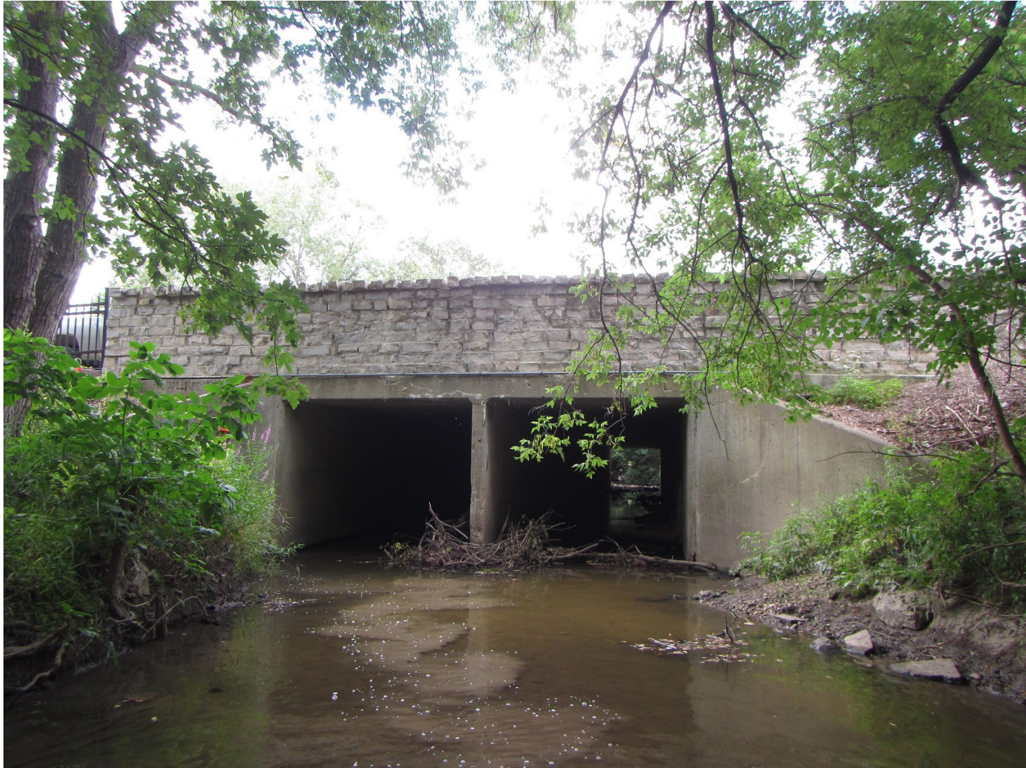
Figure 11: Existing culvert north elevation
