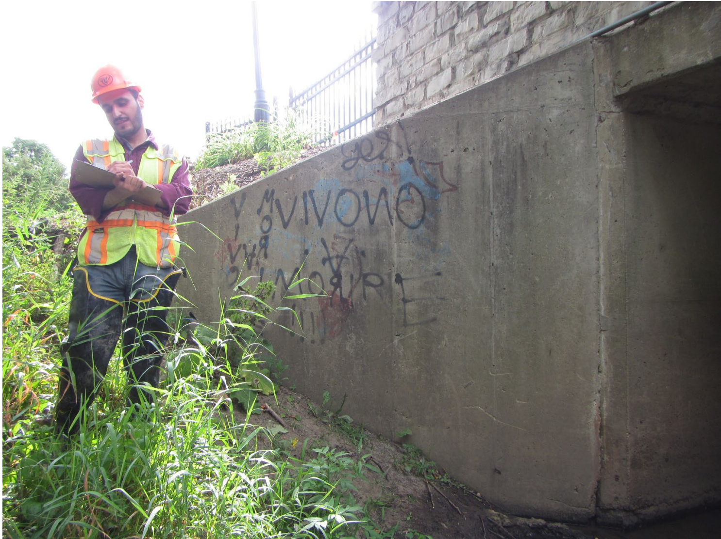
Figure 13: Existing culvert northeast wingwall
