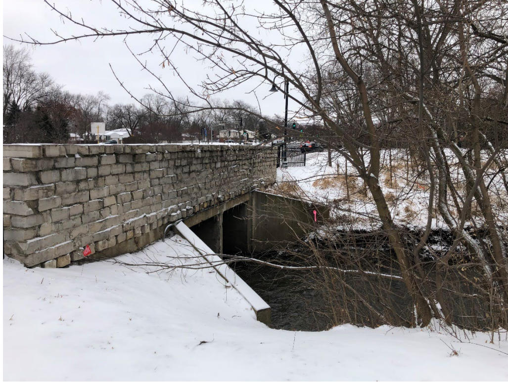
Figure 17: Existing culvert south end, looking east
