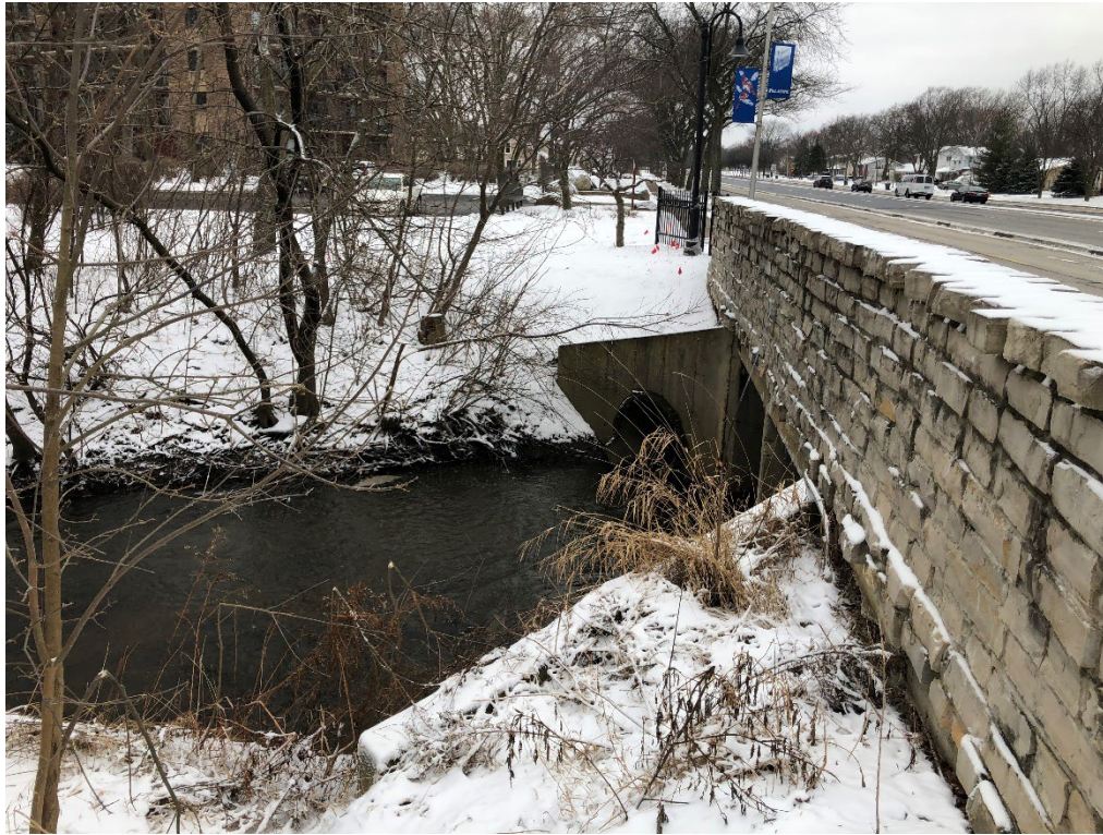
Figure 18: Existing culvert south end, looking west
