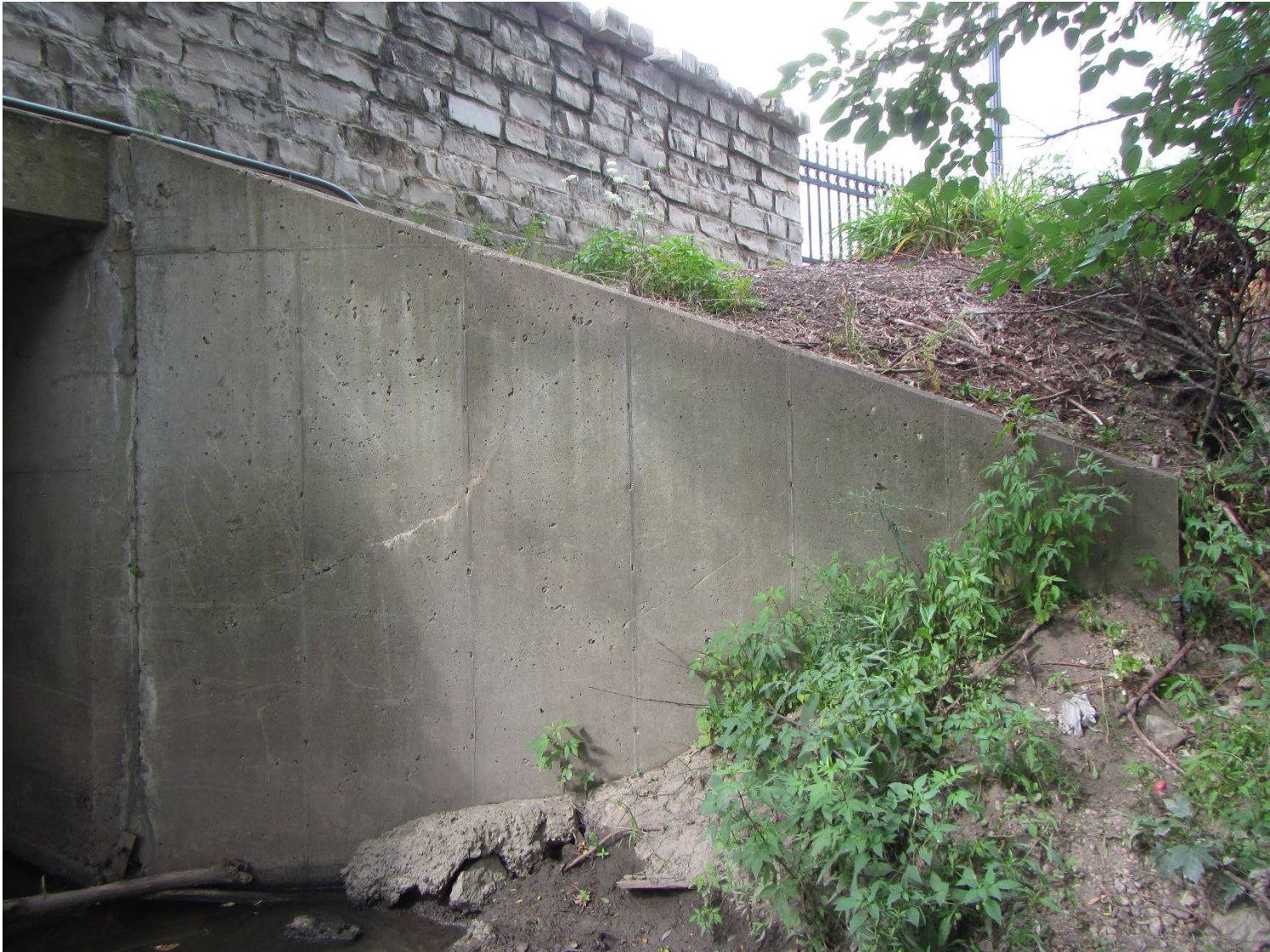
Figure 9: Existing culvert northwest wingwall
