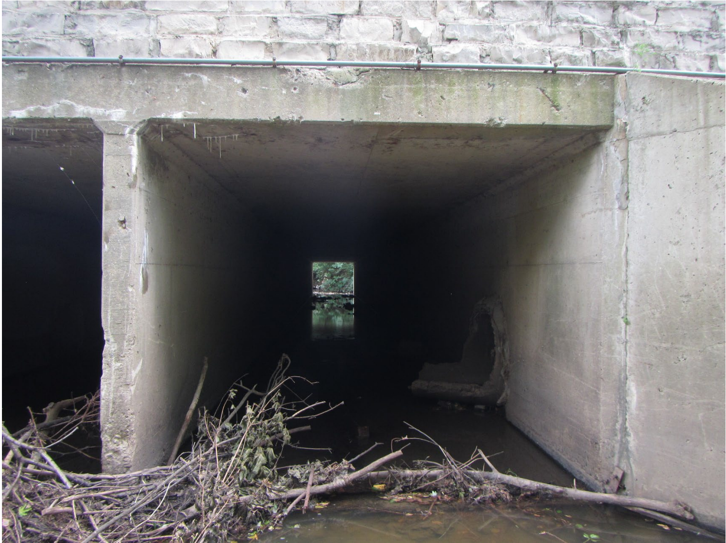
Figure 14: Existing culvert north headwall (cell 1)
