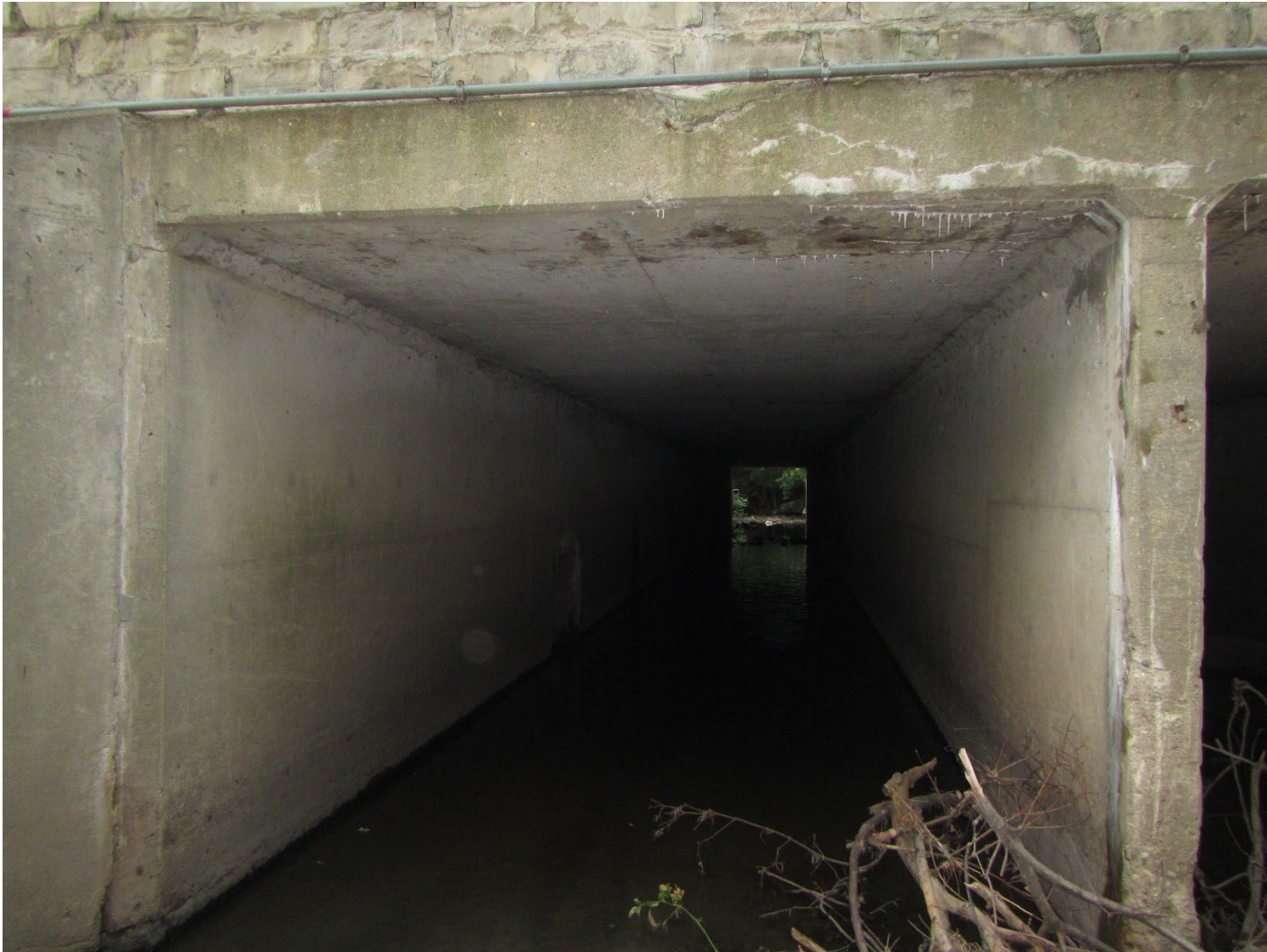
Figure 15: Existing culvert north headwall (cell 2)
