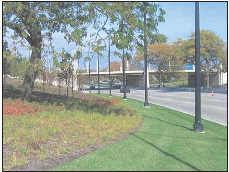
South Lakeshore Drive Reconstruction - 59th Street Underpass
