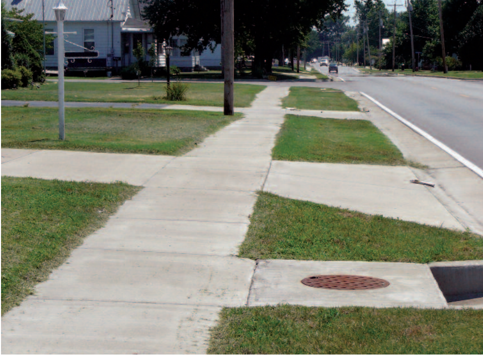
Sidewalk running slope and cross slope should continue through commercial or residential driveways
