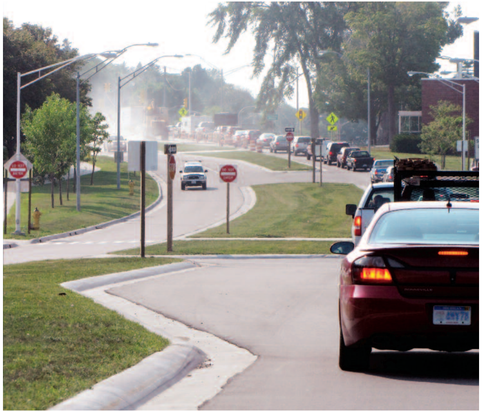
Dedicated turn lanes, pedestrian refuge areas, adequate signage, and wide separation between traffic lanes all contribute to the safety of a road. The new Highway Safety Manual provides guidance for determining the best treatments to address safety concerns.
