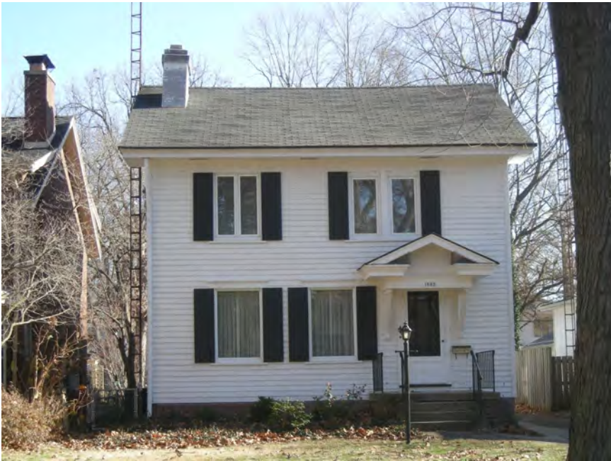
Figure 3: 1532 S. Noble Ave., camera facing east (12-14-2009)
