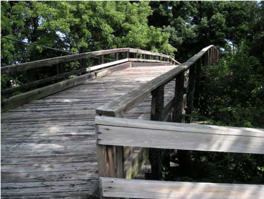
Timber Stringer bridge
