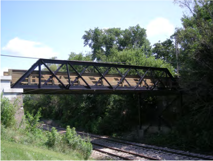
Steel Truss, Quadrangular Warren bridge
