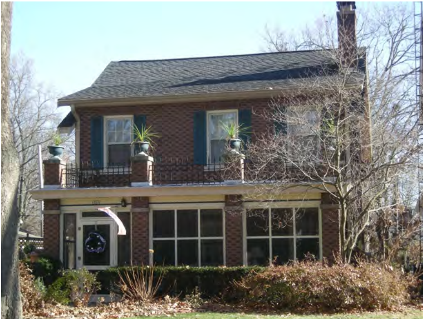
Figure 4: 1528 S. Noble Ave., camera facing east (12-14-2009)
