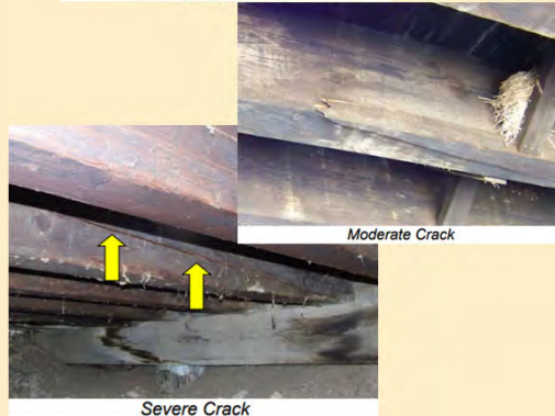
Severe Crack
