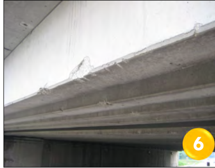
No beams with reinforcement exposed at center span
