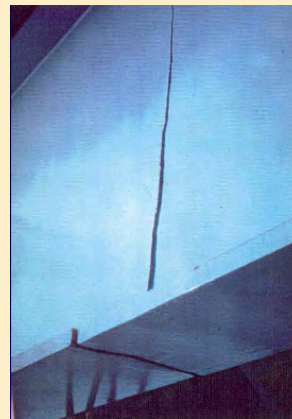
Fractured Girder
