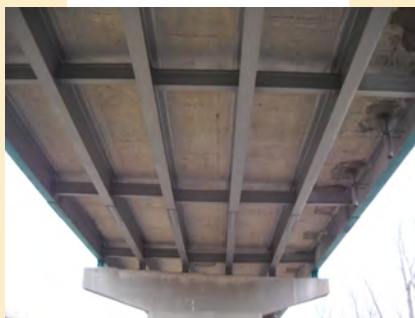
Load Path Redundant
