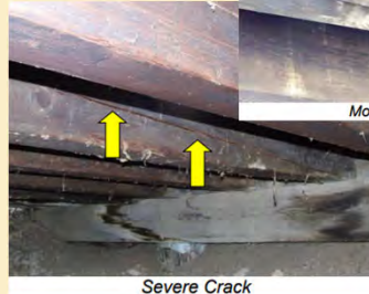
Severe Crack
